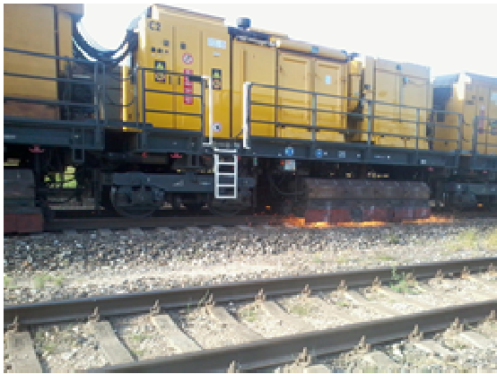
Fig. 1. Grinding of 1st main track in station Taurkalne with “Speno” rail grinder
